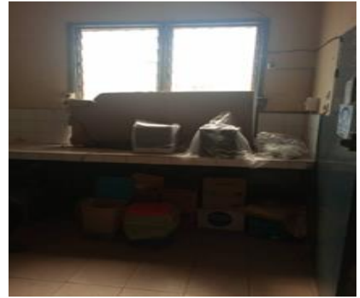
Gene Xpert Unit before renovation
